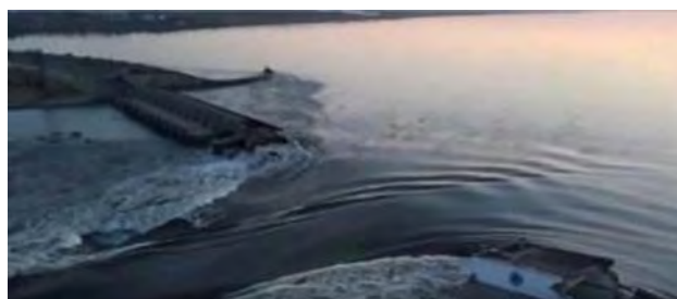
Figure 29 Kakhovka Dam destruction
